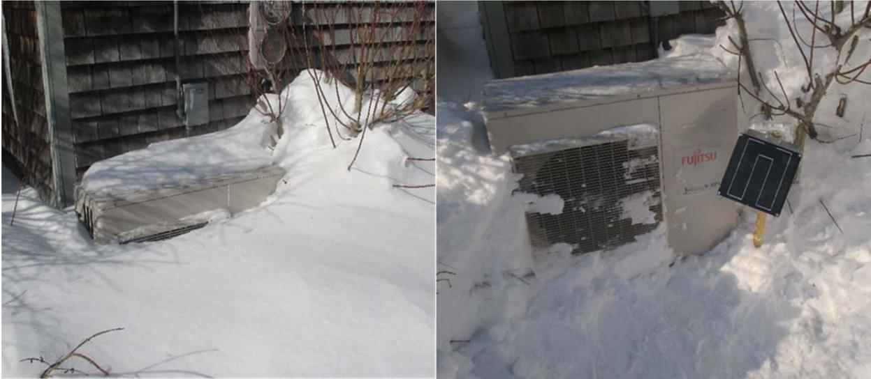
The direction and presence of significant, prevailing winds also can play a role in outdoor unit performance. At an oceanfront site examined during the study, the DMSHP outdoor units were directly exposed to a strong ocean breeze. During summer, this unit placement boosted performance as the ocean breeze helped draw heat out of the unit and aid in the cooling process.
