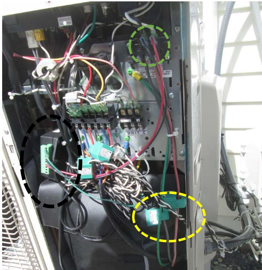
The watt-hour transducer measured voltage and current supplied to the DMSHP system and converted energy consumed during the time interval to a number of pulses. The team then used the number of pulses and the logging interval to derive average power and energy consumed over that time period.
