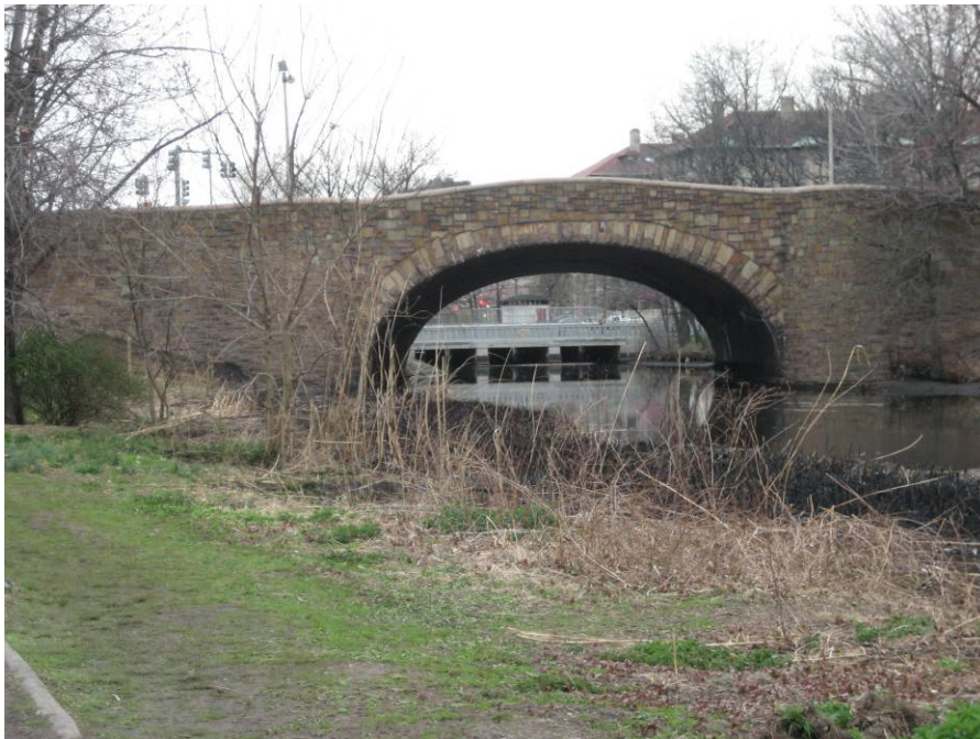
Image of Boylston Street bridge 2010 after the April wild fire.
