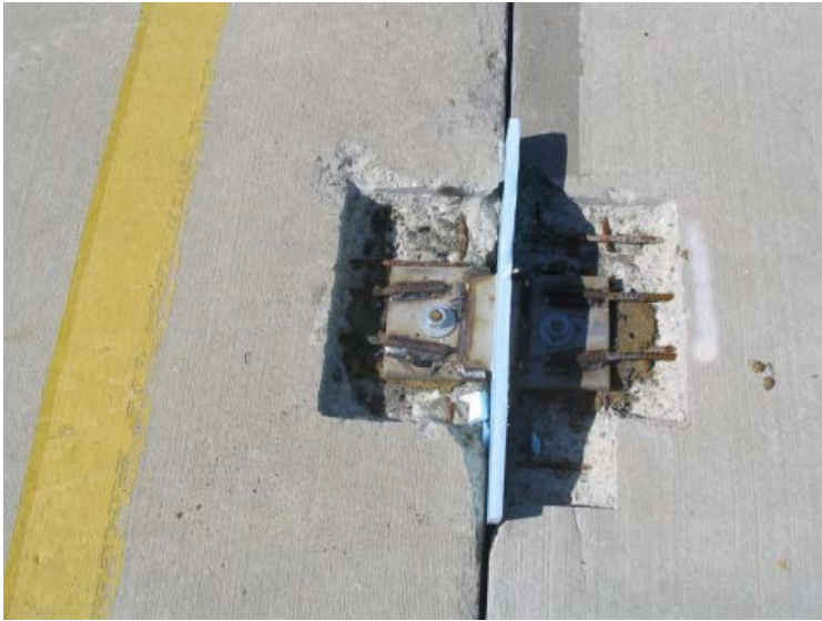
Example of Flange Connection Repair
