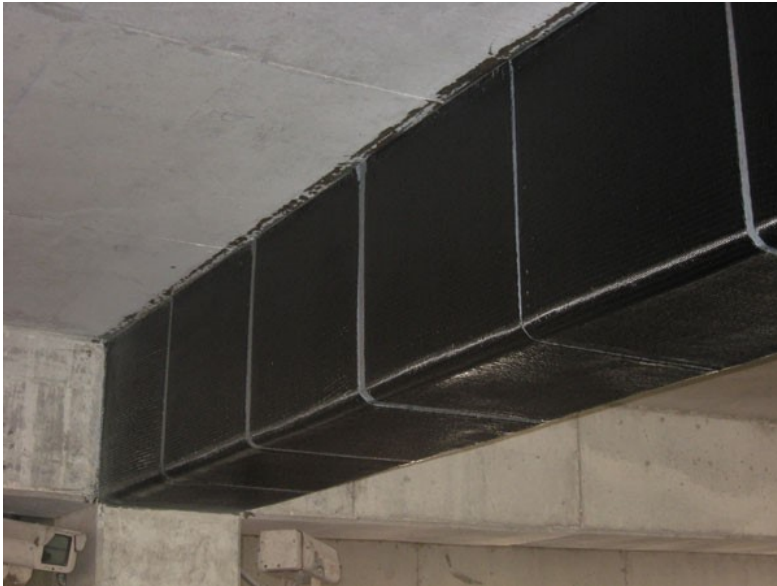
Example of Carbon Fiber Repair
