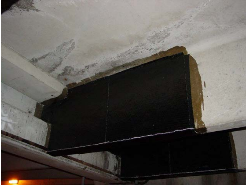
Example of Carbon Fiber Repair
