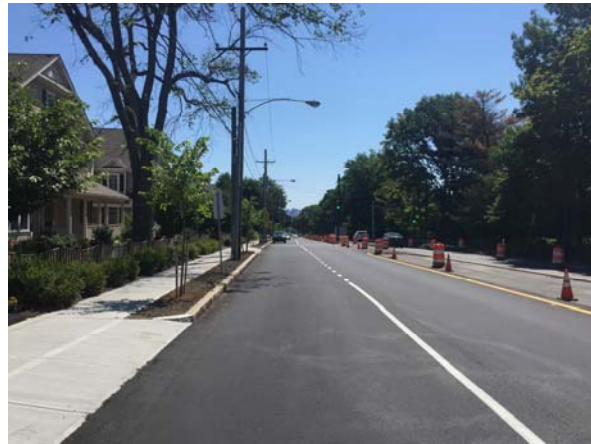
Completed Sidewalks and Intermediate Pavement Layer
