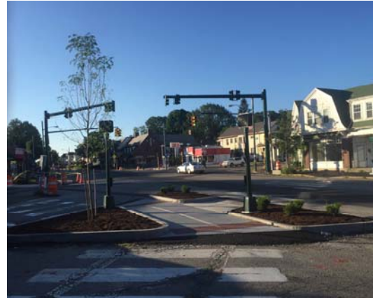
Signal and Streetscape Work at Cushing Square
