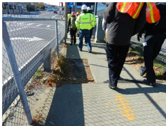
Sidewalk tripping hazards at empty tree
