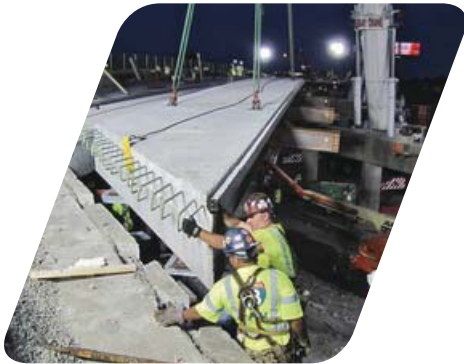
Innovation – Award-winning Fast 14 rapid bridge replacement saved millions of dollars and valuable time on I-93 by using innovative techniques – Medford
