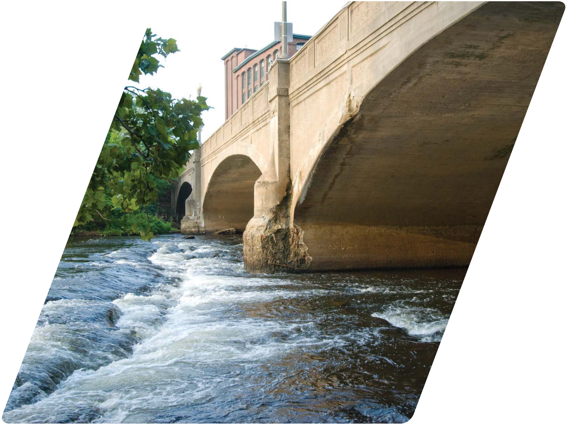
Water damaged abutments of Davitt Memorial Bridge
